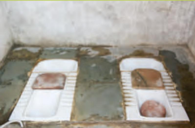
The Ecosan toilet keeps dry and wet waste separate. One pan is used until the tank below is full; the pan is then closed (right) and the other used while the collected dry waste turns to manure
